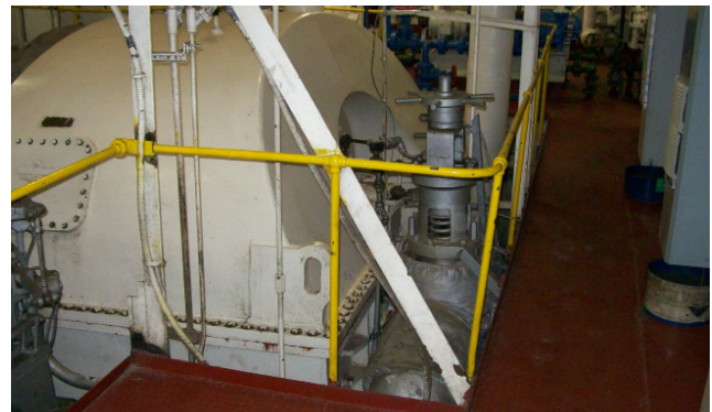
Figure 11 – Top Portion (Safety Valve) of Boiler of El Faro (Source: NTSB)
