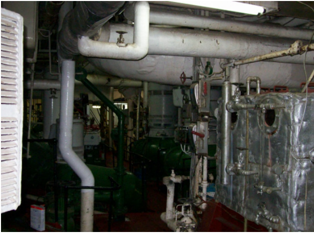
Figure 14 – Power Generation Turbines of El Faro (Source: NTSB)
